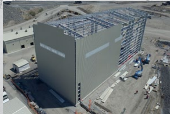
450 tons. Welding Workshop of screwed metal structure – 10.000 screws approx.
